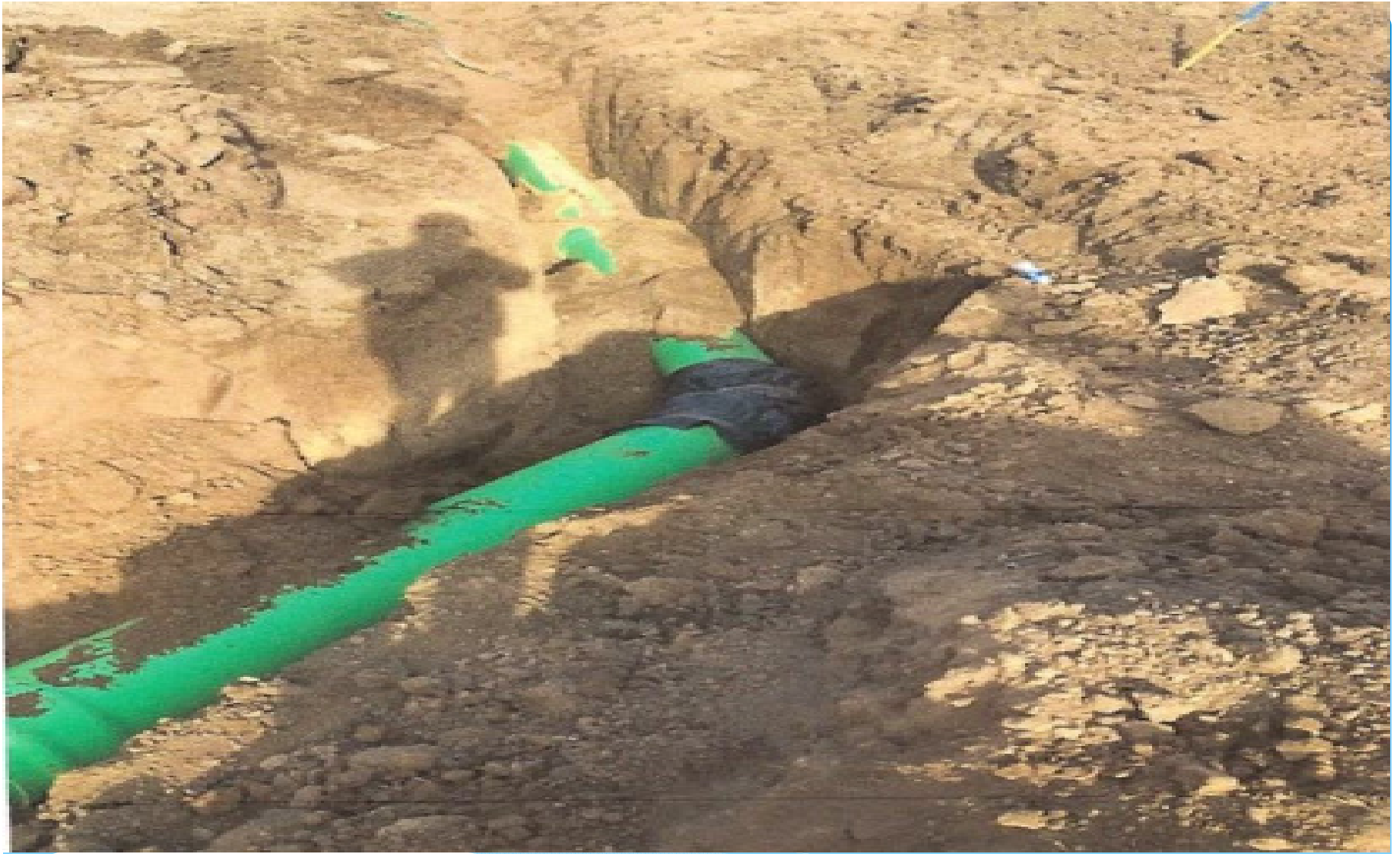
Mor-Wil Construction- Force Main Installation
