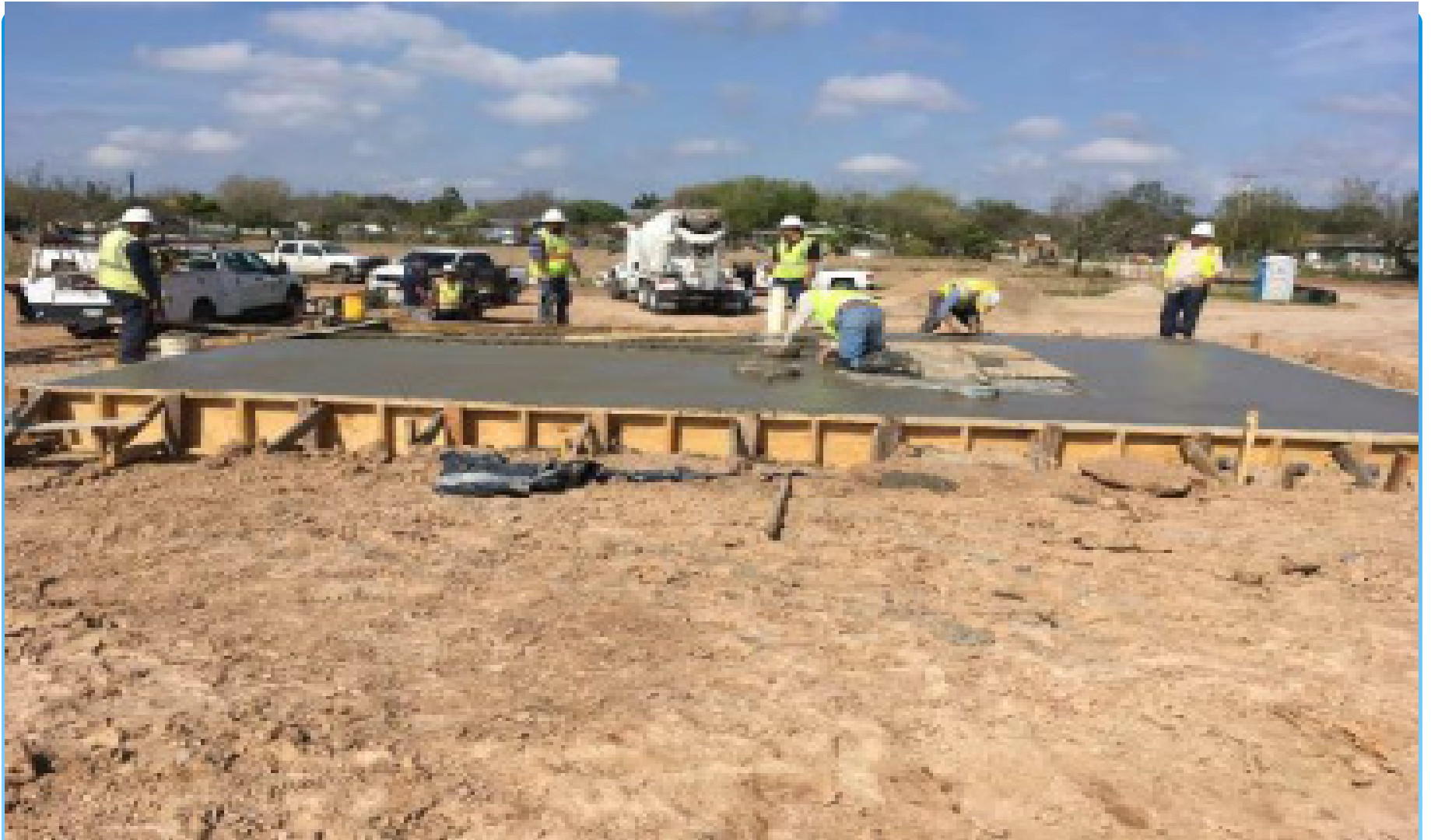
Closner Construction – LS-A2 Wet Well Concrete Pad
