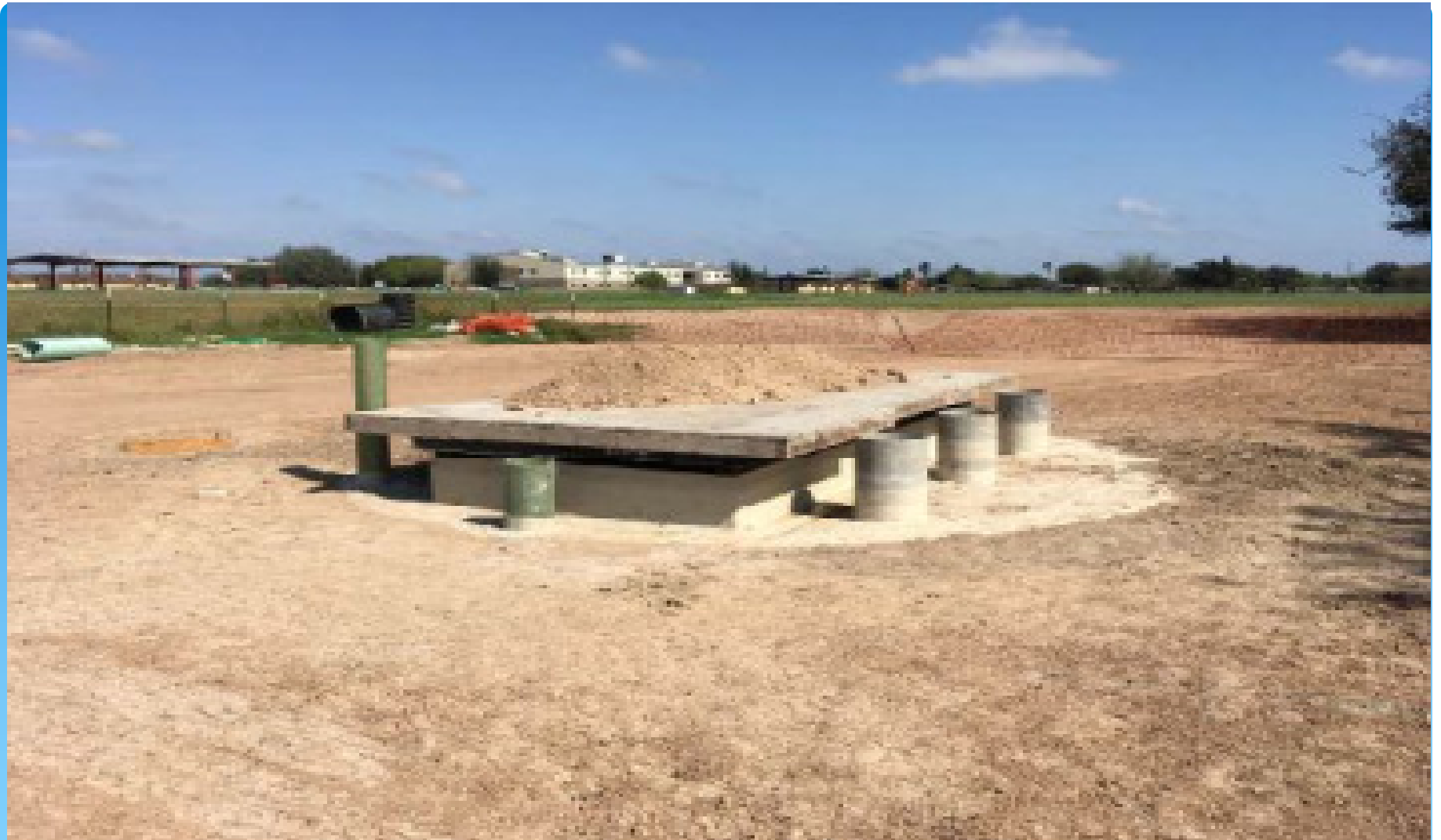
Closer Construction – Piping & Hatches at LS-F
