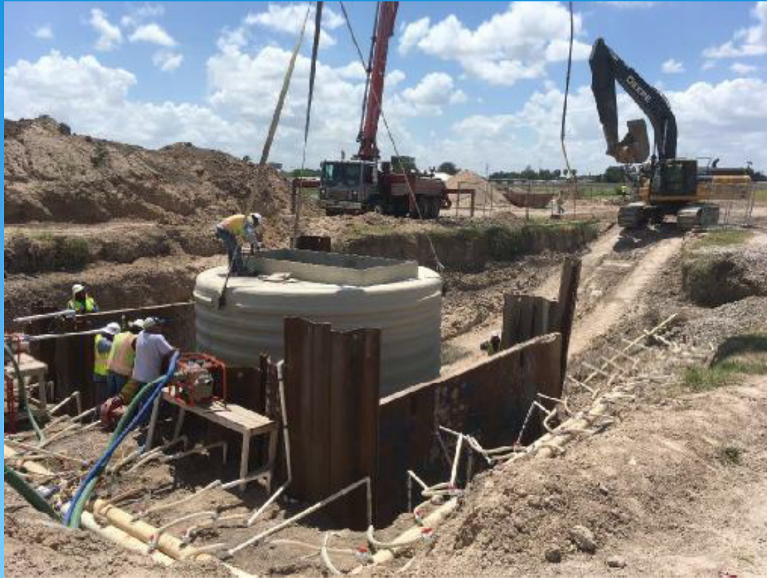
LIFT STATION 'G7' INSTALLATION OF WET WELL
