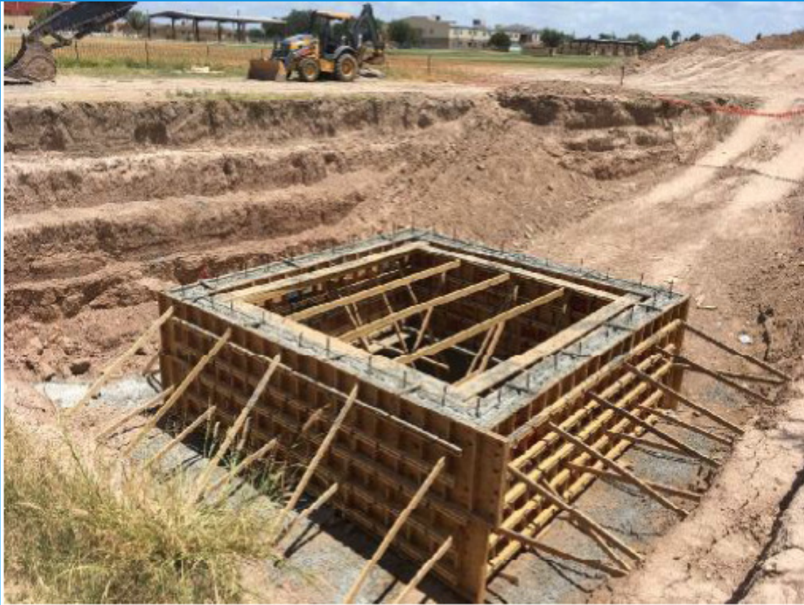
LIFT STATION 'F' CONCRETE CAISSON SHORING (2 ND 8' HIGH SECTION)
