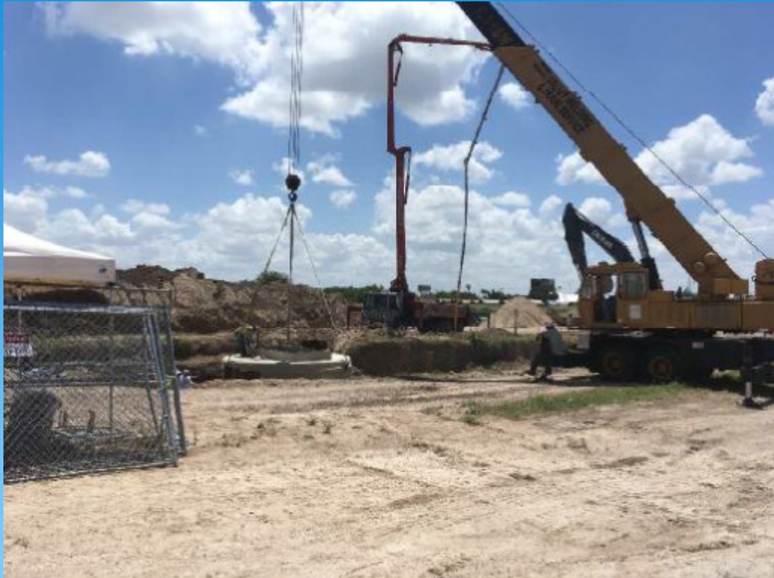
LIFT STATION 'G7' INSTALLATION OF WET WELL
