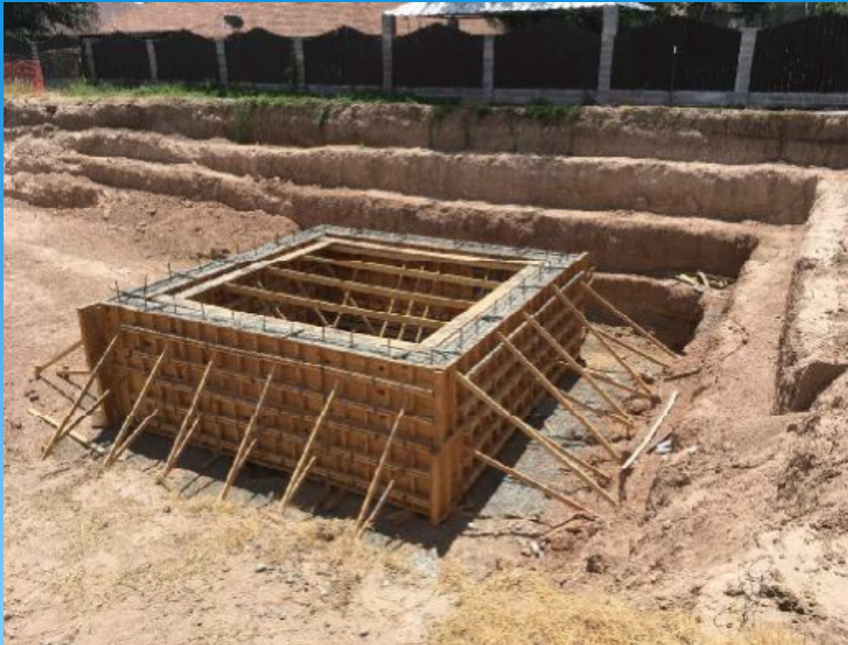
LIFT STATION 'F' CONCRETE CAISSON SHORING (2 ND 8' HIGH SECTION)
